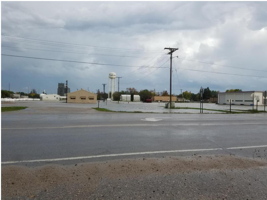
Photo 2: 2019 flooding of businesses along TH 89 due to inadequately sized storm sewer
